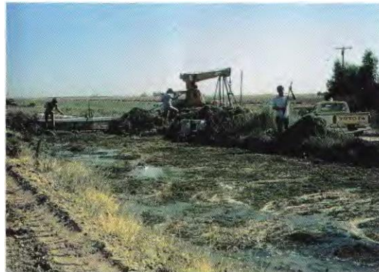
Mechanical removal of hydrilla
