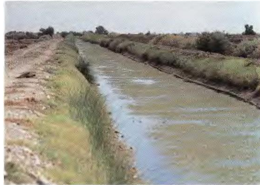
Hydrilla growth in irrigation canals can result in reduced flow and water delivery
