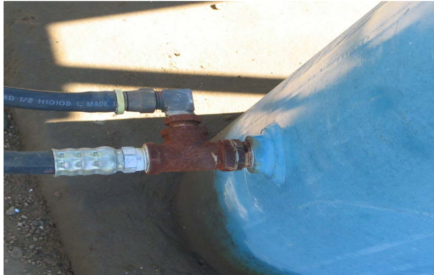
Figure 2, Hydraulic Fuel Line and Fittings. Note looping of return line at this point.
