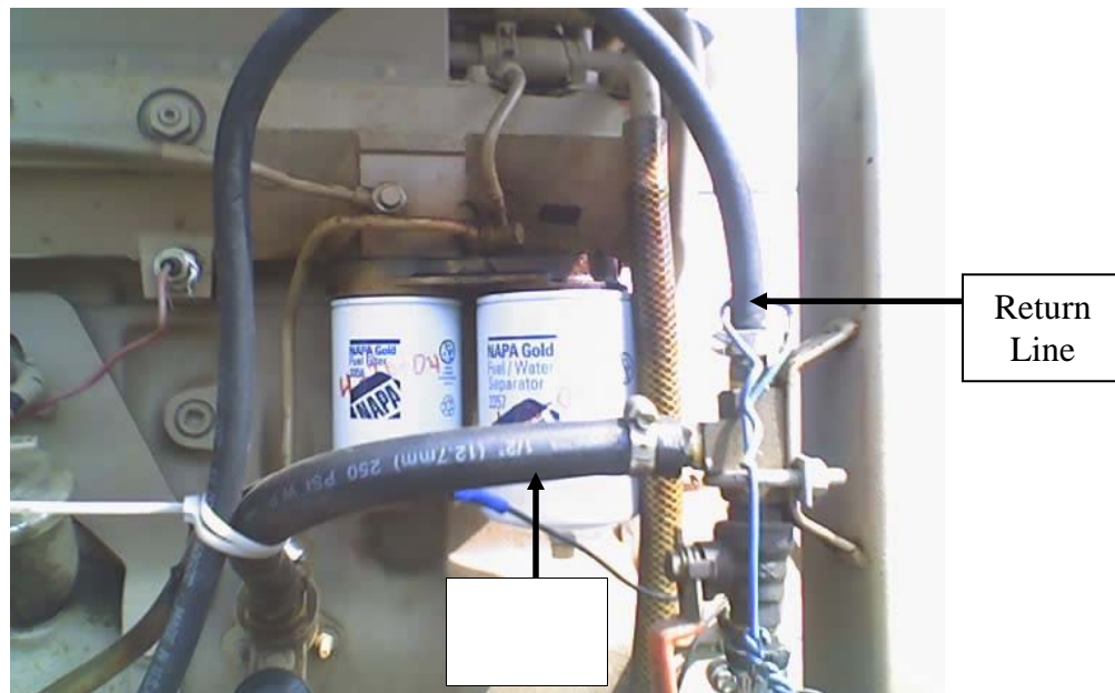
Figure 3, This engine has the return line and supply line looped at the engine. Not recommended by the engine manufacturer as there is not adequate cooling of the fuel before returning to the injectors.
