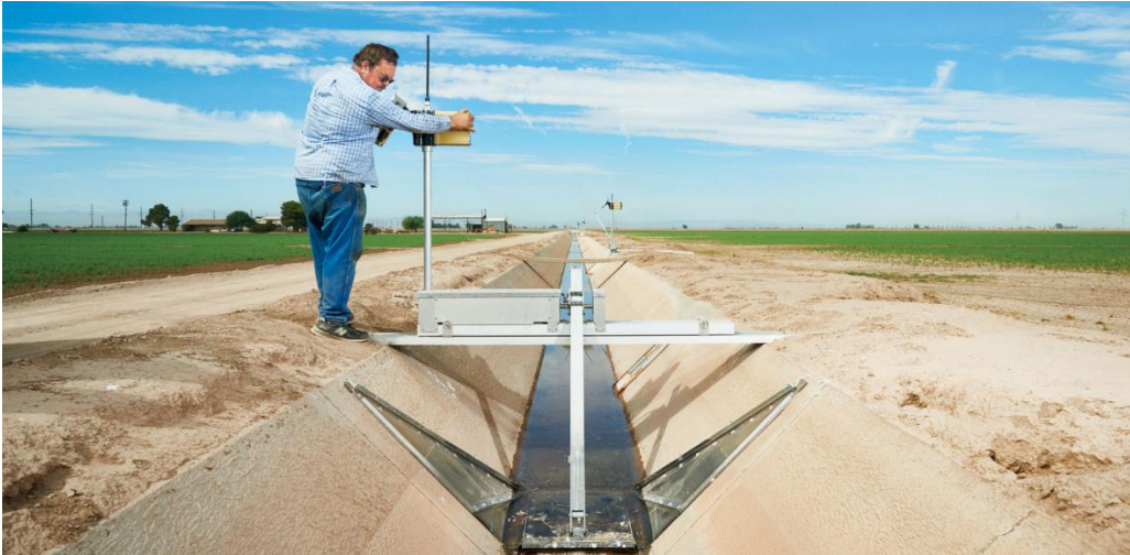
Figure 4 Example of a BayDrive actuation for farm canal at RCL Farms Holtville CA
