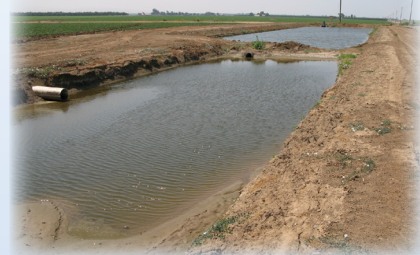
Shown above and below, holding ponds for recirculation systems in Stanislaus County. Tailwater recirculation systems facilitate the reuse of drainage water and help keep pesticide residues out of waterways. Photos: CURES
