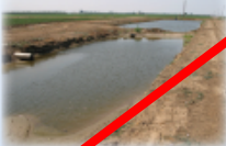
Shovel-ready and below, holding ponds for recirculation systems in Stanislaus County. Tailwater recirculation systems facilitate the reuse of drainage water and help keep pesticide residues out of waterways. Photo: CURS
