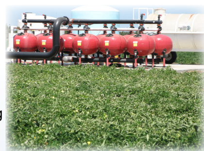
A drip system for tomatoes in Stanislaus County. Photo: CURES
