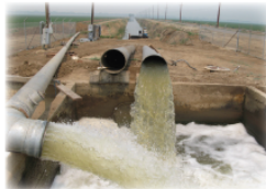
A tailwater recirculation system in Stanislaus County. Photo: CURES
