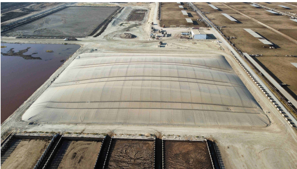
Pictured above: Bar 20 Dairy fuel cells and dairy digester funded through DDRDP
