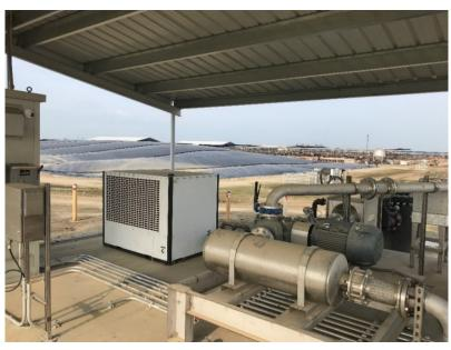
**Image 15.** Biogas conditioning equipment (foreground) and covered lagoon digester (background) at Riverview Dairy.
