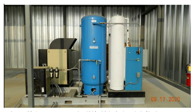
**Image 19.** An oxygen generator skid for biological control of hydrogen sulfide (H<sub>2</sub>S) at Trilogy Dairy.
