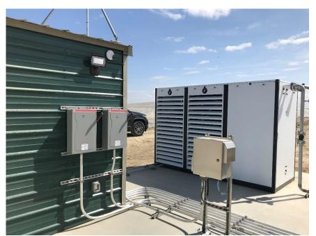
**Image 11.** Biogas conditioning equipment (foreground) and covered lagoon digester (background) at Cornerstone Dairy.
