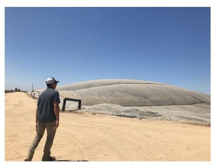
Image 14. Covered lagoon digester filled with biogas at the Vander Poel Dairy.
