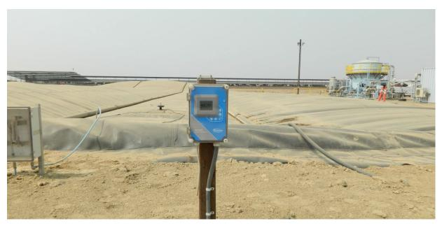
**Image 18.** Weir box and a weir box meter (foreground) and covered lagoon digester and biogas conditioning equipment (background) at Maple Dairy.
