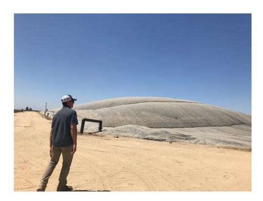
Image 12. Covered lagoon digester filled with biogas at the Vander Poel Dairy.
