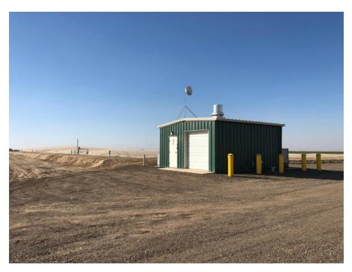
**Image 6.** View of biogas handling building (foreground) and covered lagoon digester (background) at Circle A dairy.
