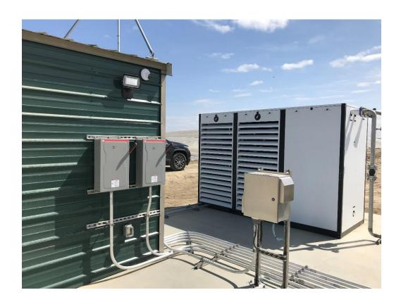
**Image 9.** Biogas conditioning equipment (foreground) and covered lagoon digester (background) at Cornerstone Dairy.
