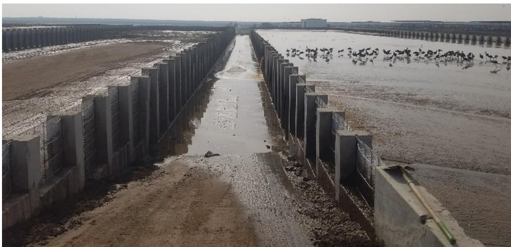
Figure 5. Dairy E: Weeping wall, a view of 2 adjacent cells The left cell is empty while the right cell is filling
