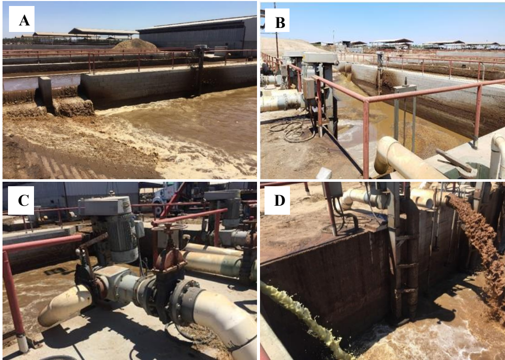
Figure 23. Dairy B: (A) flush manure from sand trap into reception pit, (B) reception pit, (C) separator pump, and (D) flush manure and milk parlor process water into reception pit
