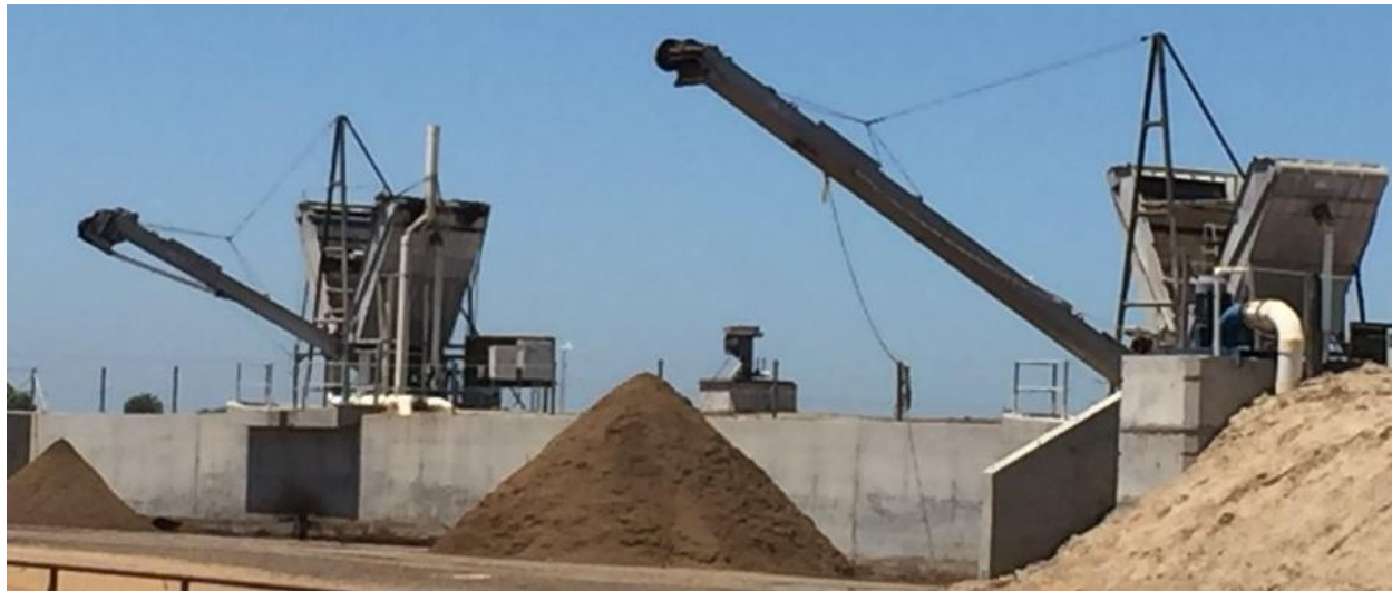
Figure 2. Dairy B: 2-stage sloped dual-screen separator as seen from the processing pit
