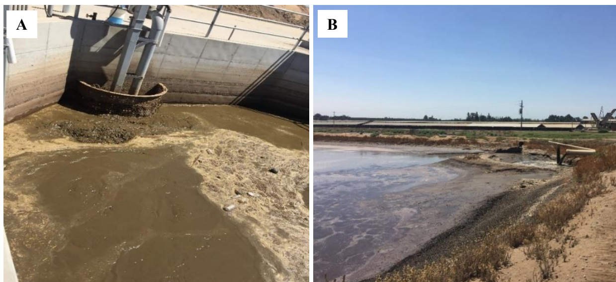
Figure 12. Dairy A: (A) flush pump in the reception pit, and (B) separator outflow into the first storage lagoon
