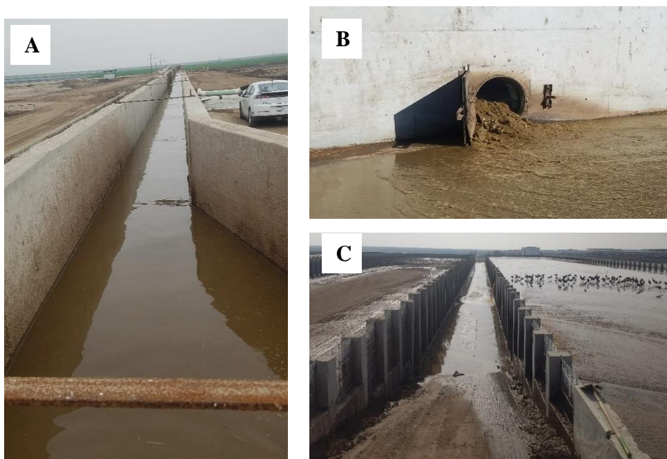
Figure 52. Dairy E: (A) flush manure receiving wall, (B) 24” valve out of receiving wall, and (C) weeping wall cells, right one filling and left one being emptied.
