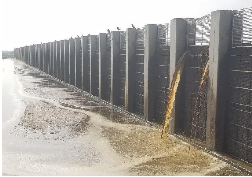
Figure 6. Dairy E: Weeping wall weeping during a cell filling
