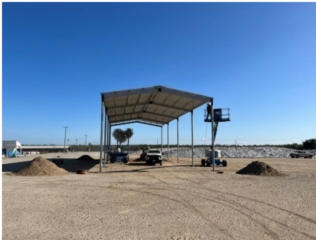
Construction of metal building for the pelletizing equipment.
