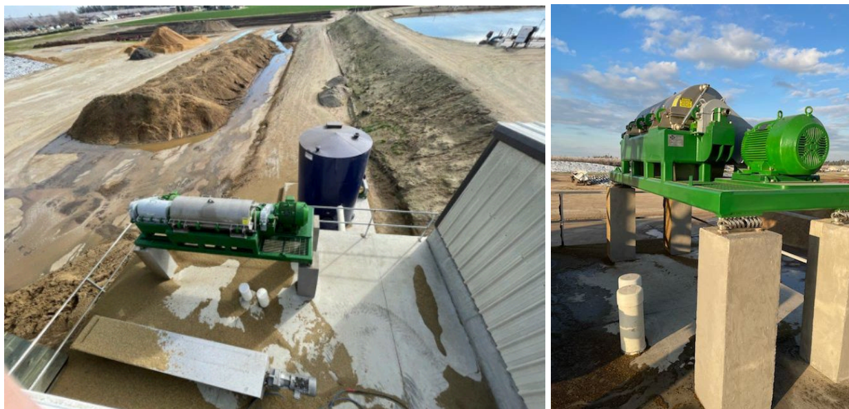
Aerial picture of centrifuge system including concrete pads, centrifuge, auger, and feed tank (left); close up of centrifuge and concrete riser pillars (right).
