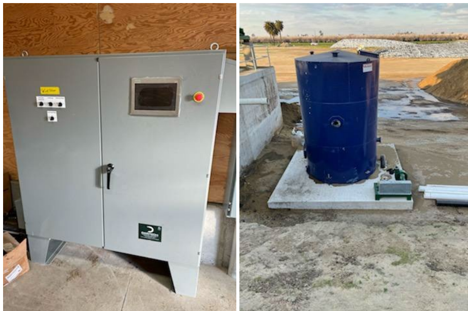
Electrical centrifuge control panel (left) and metal feed tank and concrete pad for the centrifuge (right).
