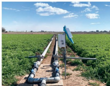
Figure 2. Magnetic flow meters and data store and transfer equipment monitors water applied to a 2022-23 field trial.
