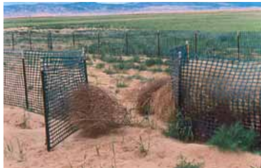
Figure 9: Porous wind fences are commercially available. They trap blowing tumbleweeds as well as sand. In areas with endangered species, such as the desert tortoise, openings should be provided at intervals to allow for continued natural migration of the animals.
