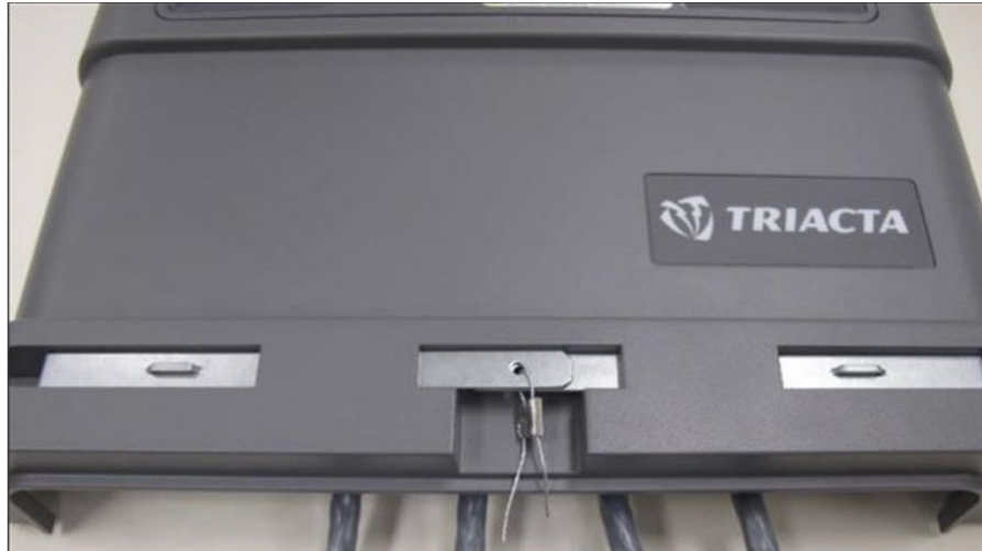
Figure 3. Category 1 wire terminal block sealing location example.
