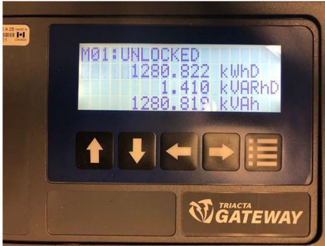
Figure 6. Showing an example of the UNLOCKED condition that needs to change prior to sealing.
