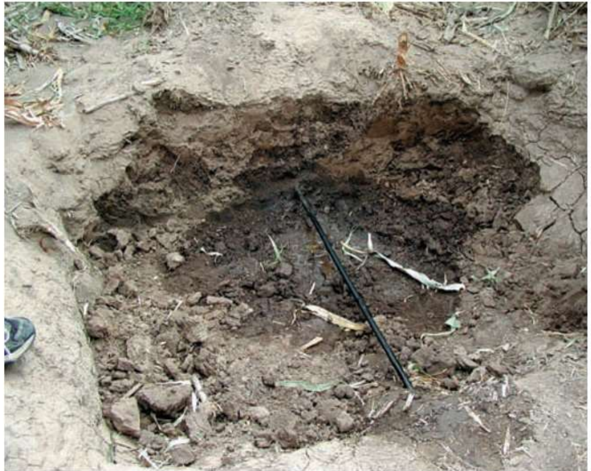
Figure 1. Dripline installed underground.
