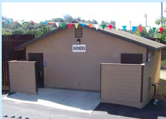
A new restroom with showers at the Mariposa County Fairgrounds. Shower facilities are an important feature for fairs being utilized as emergency staging areas.
