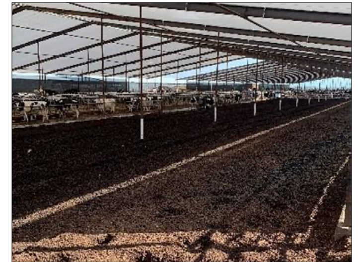
Compost Bedded Pack Barn installed for a 2017 AMMP project.
