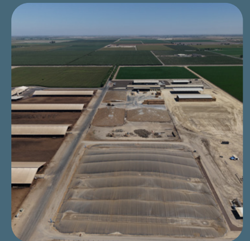
Aerial views of lagoon with liner.
