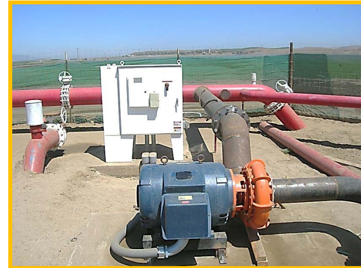
New Electric Booster Pump
