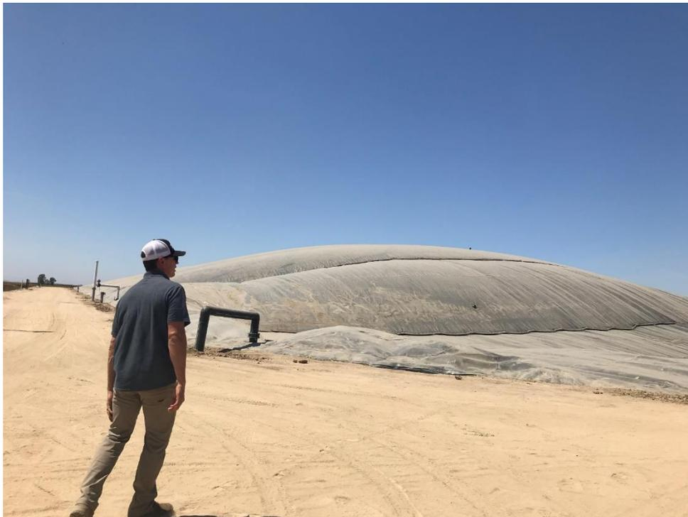
**Image 12.** Covered lagoon digester filled with biogas at the Vander Poel Dairy.
