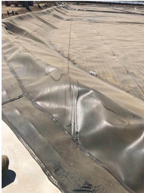
**Image 10.** Details of the digester lagoon cover at K&M Visser Dairy showing details of welded liners to prevent biogas leakage.
