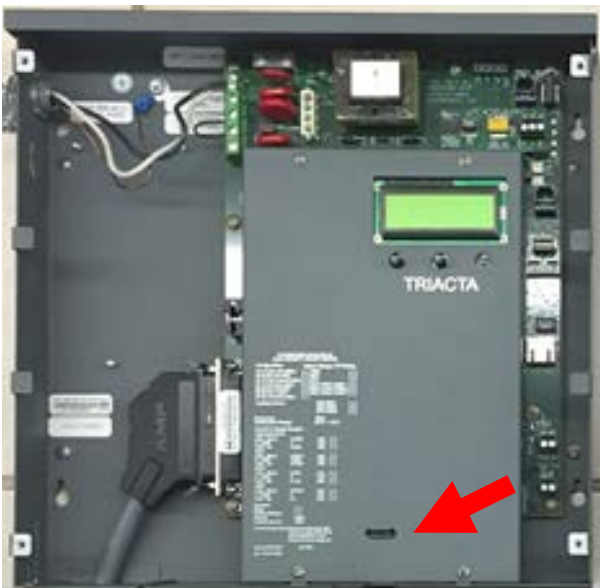
Figure 5. The printed circuit board (PCB) cover (meter seal) utilizes a physical wire security seal sealing provision. The red arrow points to the location of where the wire security seal needs to be.
